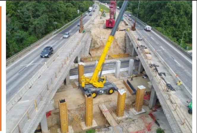
Median work on I-64
