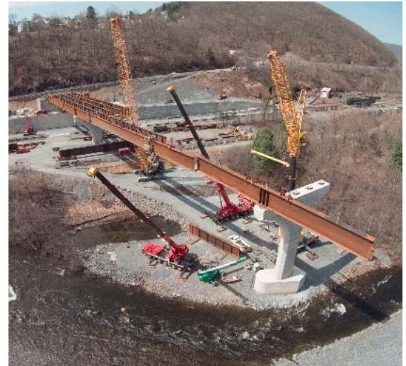
Figure 3.5.3 Causeway for the new Lehigh River Bridge in Jim Thorpe, PA
