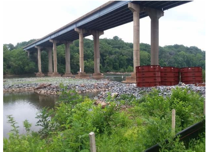
Figure 3.5.2 I-95 SB Project Causeway
