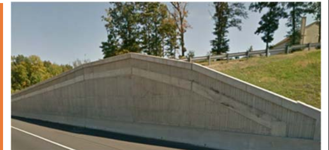
Maintenance of Traffic along I-95
