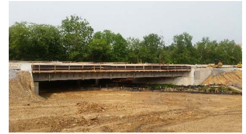
Bridge over Little Tuckahoe Creek
