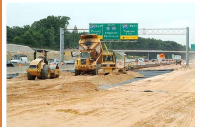
Fill placement for roadway widening along I-95
