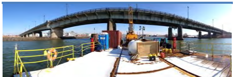
Exhibit 4.4.4.b. Barge-Mounted Geotechnical Exploration
