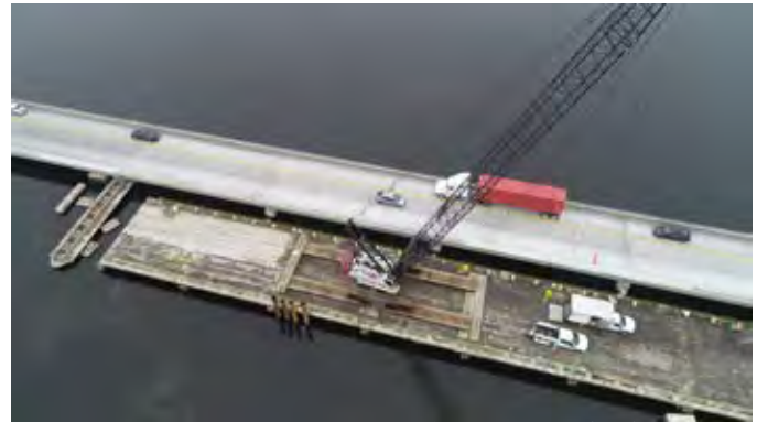
Figure 4.5.1.1: DBT reconstruction from existing bridge EFLHD Rte. 105 Lee Hall Reservoir
