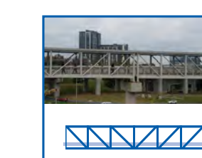
Bridge Type Tysons-Style Truss
